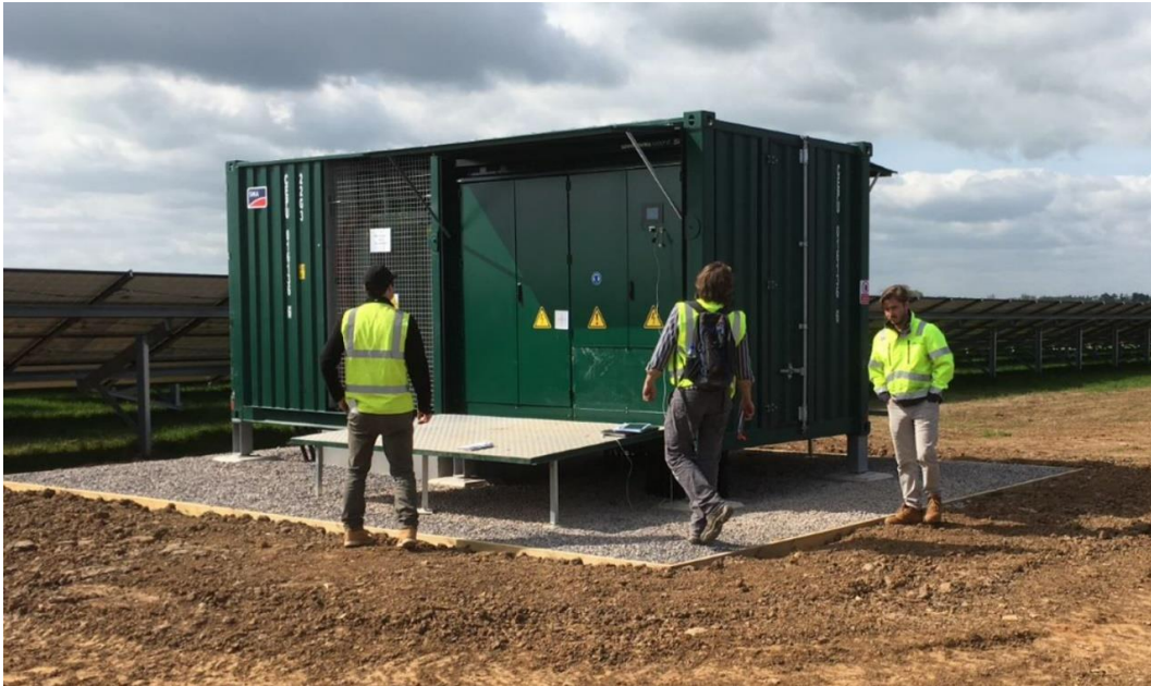
Image 3.2 – Example Centralised Inverter / Transformer Station
